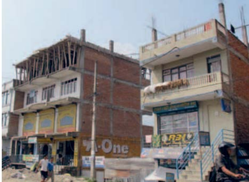
Figure 3.2. Incremental construction of an RC framed building with masonry infill walls 3
