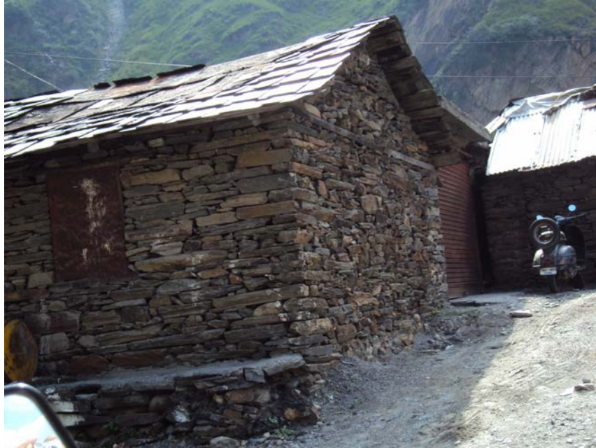
Figure 6.31. Example of uncoursed rubble stone masonry building
