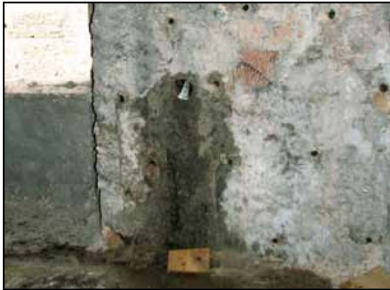
Figure 6.20. Masonry wall prepared for grout injection
