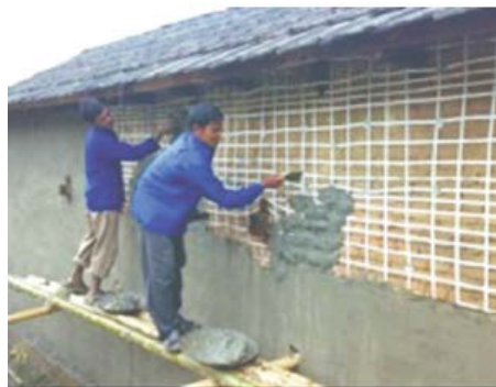
Figure 6.12. Retrofit of a house with polypropylene strips
