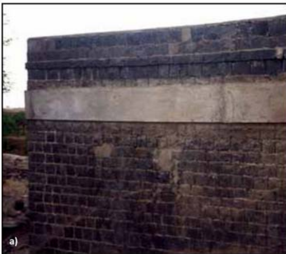
Figure 6.14. Reinforced concrete tie bands 4
