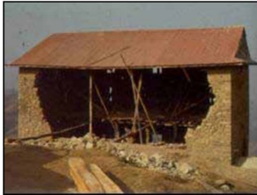
Figure 6.18. Out-of-plane failure of a stone masonry wall
