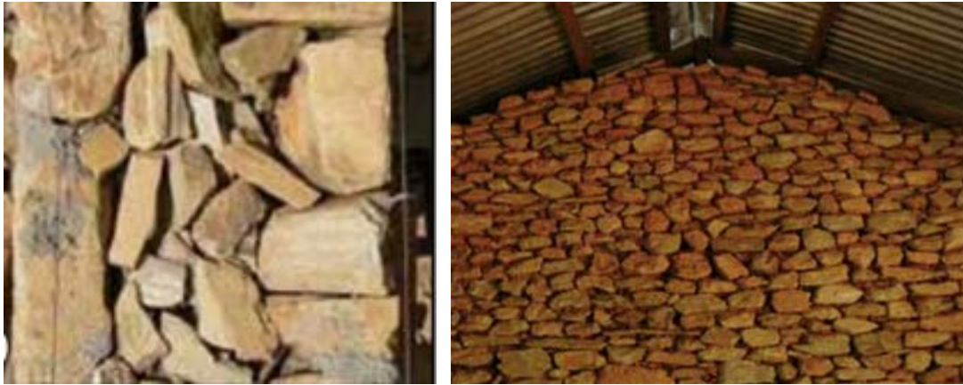
Figure 3.5. a) Cross section of a double-wythe wall and b) gable wall made of stone 4
