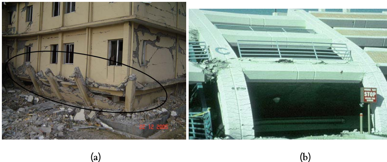
Figure 6.21. Failure of (a) non-ductile vs. (b) ductile RC framed buildings
